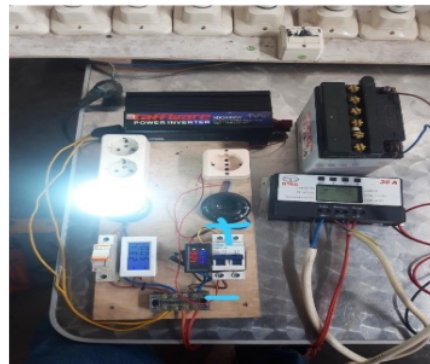
Figure 8. Test circuit using DC MCB and AC MCB with Voltage and Current Meters
