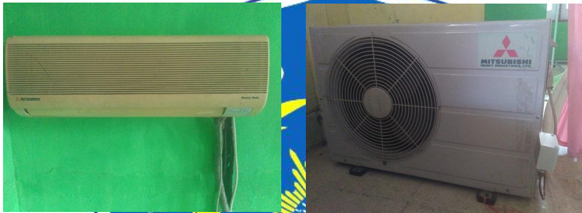
Gambar 4.4. Pengujian modul unit Air Condition (AC).
