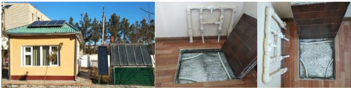
Figure 1.1. An overview of the experiment solar house and water heated floor system.
