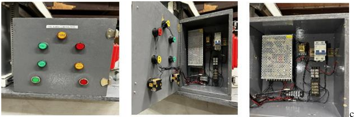
Inside wiring of modern fire alarm panel
