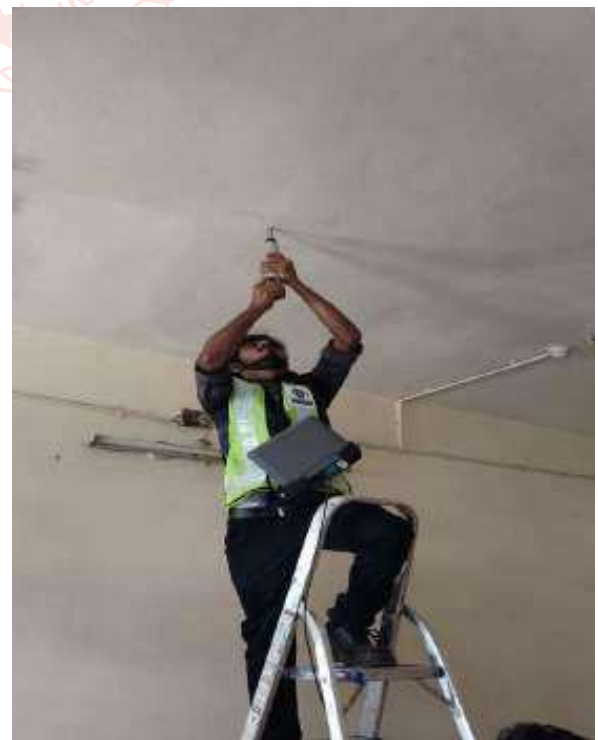
Rebound Hammer Test
